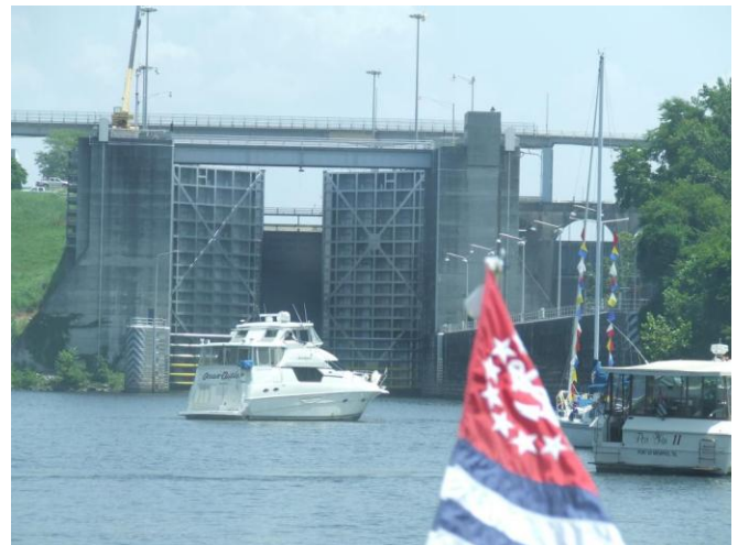
Tim Robertson and Ginger Coleman’s boat, “Ocean’s Outlaw”, enters the Wilson Lock. This is the second highest lock in the United States and the highest single lock east of the Rockies. The lift is 93-100 feet, depending on water levels.
