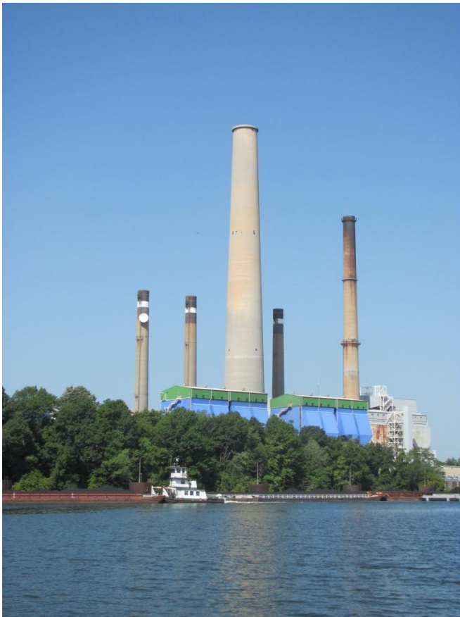
We passed close by this coal fired generating plant.
