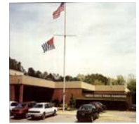
National Headquarters Raleigh, North Carolina
