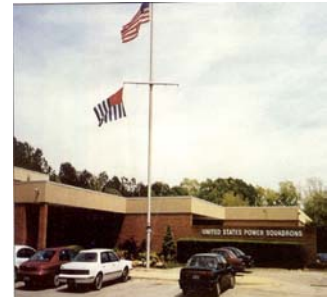
National Headquarters Raleigh, North Carolina
